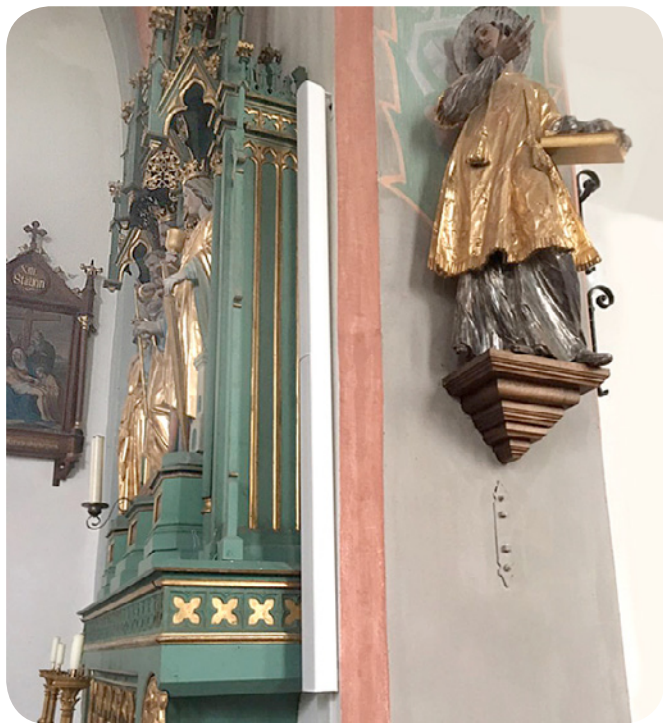
Fig.: Mounting example with K1-90 sound columns.
